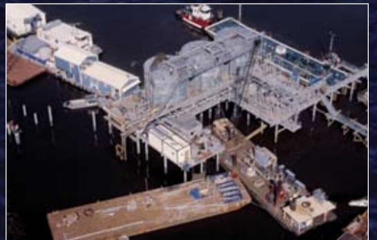
The 185-foot DSV Stephanie Morrison 's double deck configuration allows for support equipment, diving chambers, compressors and bells to be stored on the lower deck, leaving the upper deck free for materials and fabrication.
